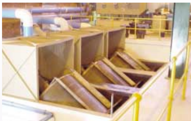
Ro2/0.5mm screen installed at a STP in Sth Africa
